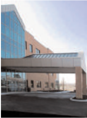
Daylighting (credit EQ 8.1) is an important consideration for orientation of the building.
