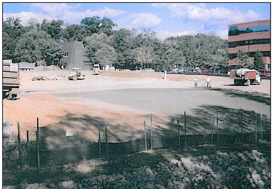
Cafferty's remediation completion-seeding and final grading.
