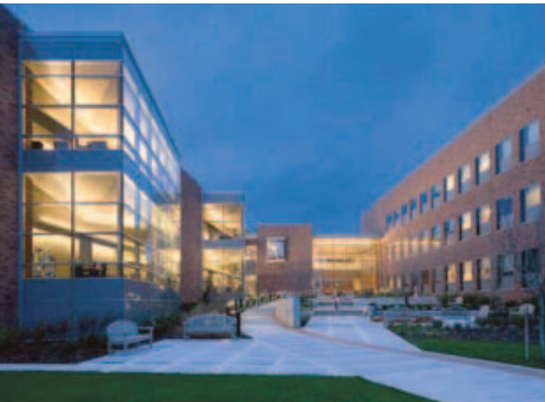
Providence Health System and Services in Newberg, Oregon—the only LEED Gold healthcare facility in the United States. Certification was awarded in August 2006.
